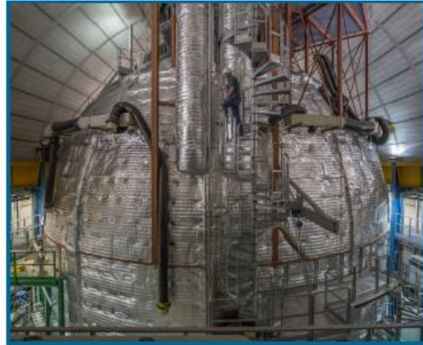
After thermal insulation
