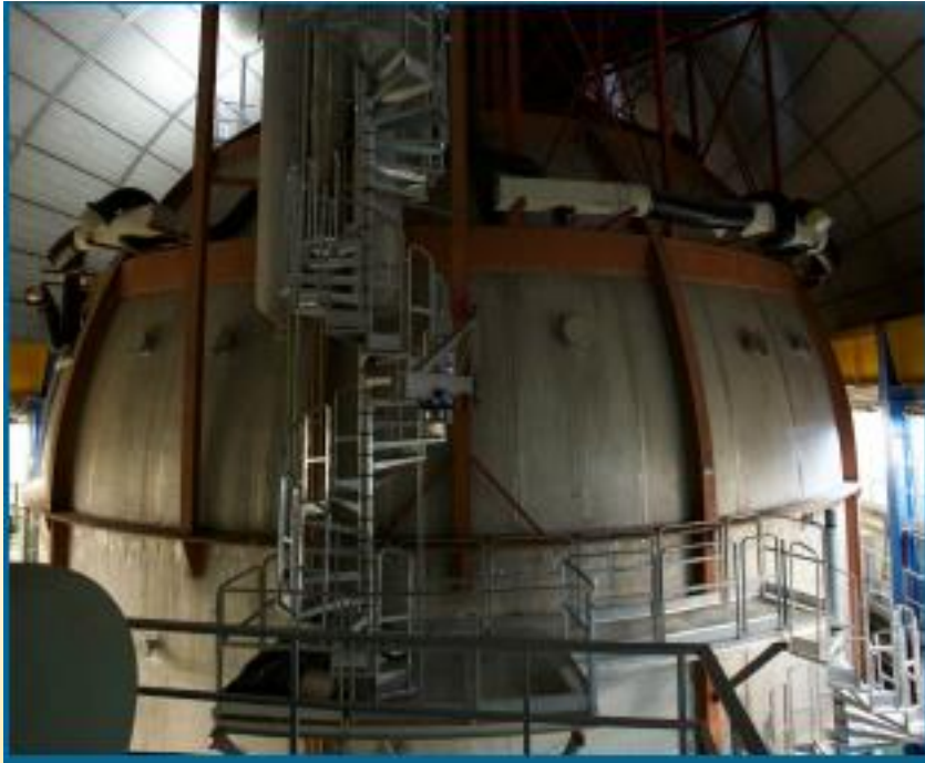
Before thermal insulation
