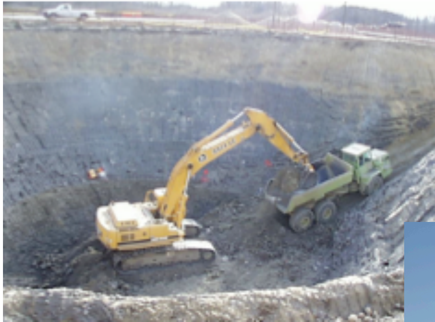
Start of construction
